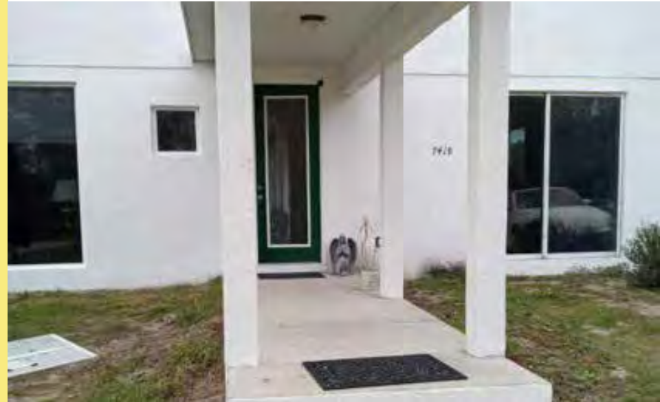
(Top) The rebuilt forest walkway/bridge. (Bottom) The staff house received essential upkeep.
